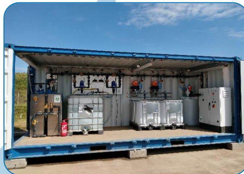
full-scale remediation with custom-made remediation units
