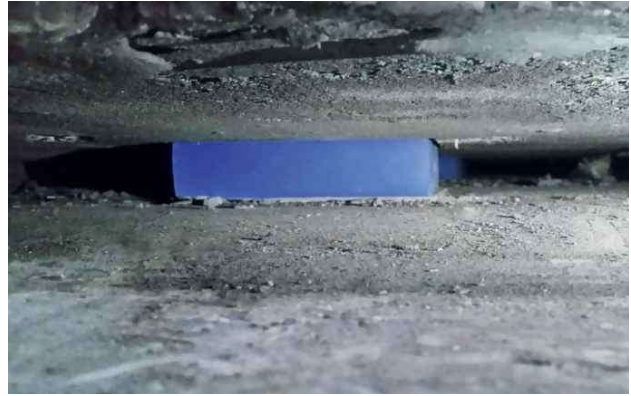
Mass-spring system with Sylodyn® discrete bearings
