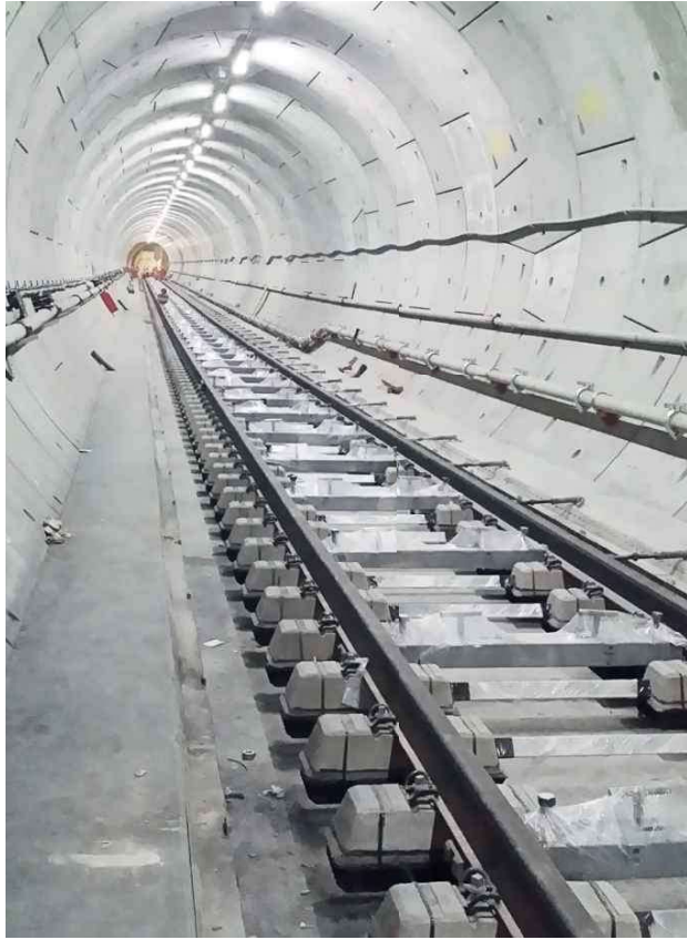
Slab track system in the tunnels
