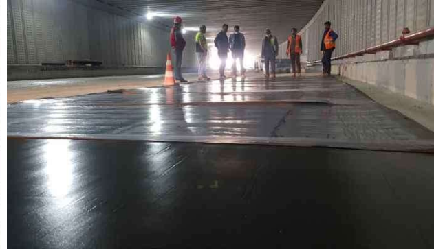
Fig 2: Mass-spring system Source: Getzner Werkstoffe
